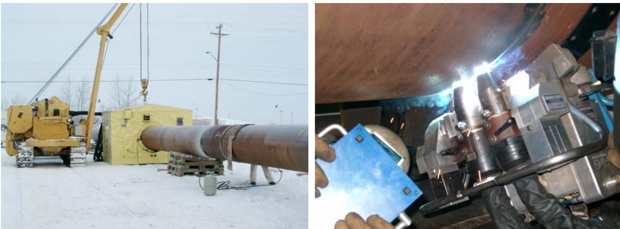
Fig. 8: Application in the area of pipeline construction. The pipelines are welded at very extreme temperatures. Reduction by a factor of 12 in the processing time per joint.
